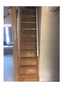
The current construction utilizes a ladder to access the main sleeping area (loft). This ladder does not meet current access regulations, and is a hazard to those who use it. The proposed works will remove the ladder and cupboards, to be replaced with a new staircase. This stair will provide safe and easy access between the main sleeping area and the living/kitchen/bath areas.
